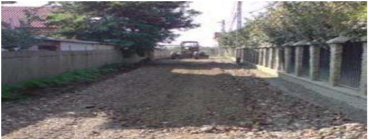
Fig. 3.2 – Demolition process and crushing of demolished material
