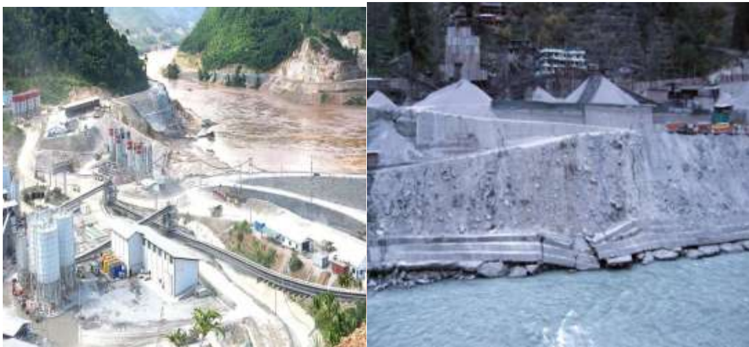
Figure 6: Damages in Hydro Power Project
