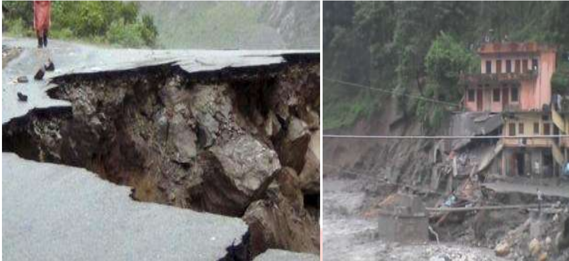
Figure 4: Damages in Uttarkashi District
