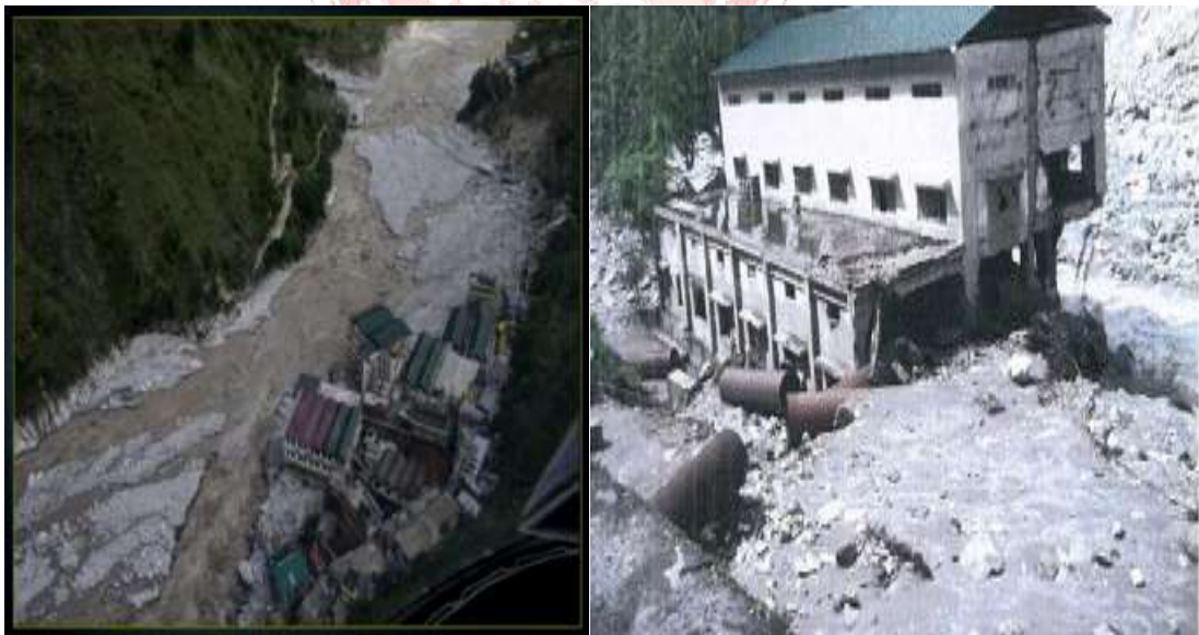
Figure 3: Damages in Rudraprayag Uttarkashi:
