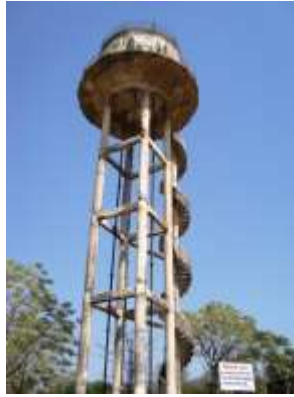
Fig. 1. Elevated Storage Reservoir
