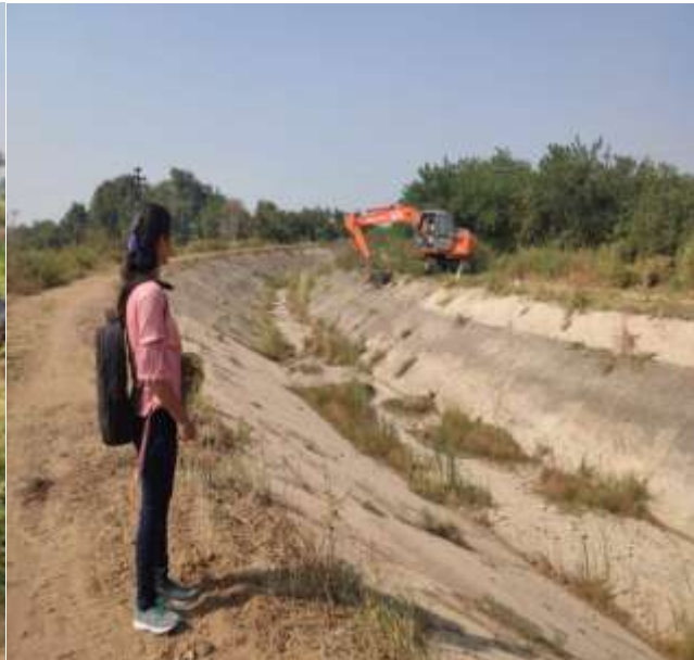
Maintenance Of Branch Canal
